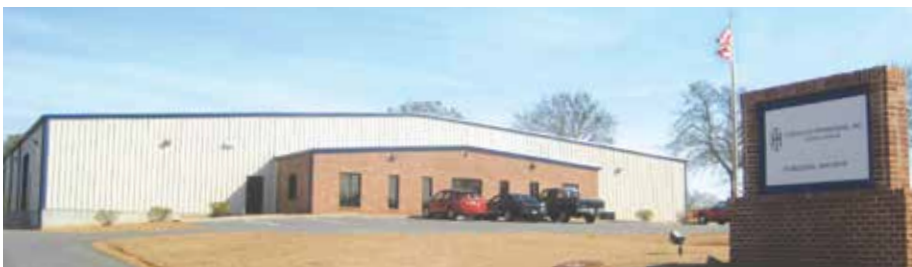
AIRCRAFT COMPONENTS AND GSE MRO FACILITY
